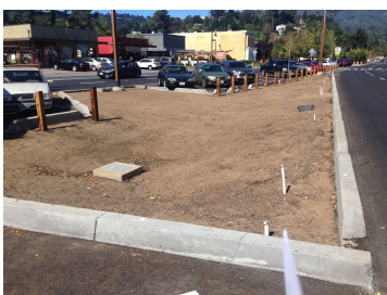
Work on Miller Avenue's rain garden.
