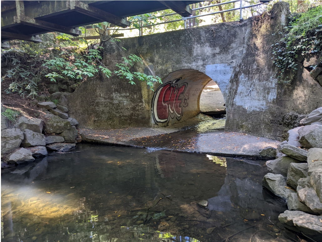
Looking upstream to culvert outfall with sloped concrete apron and plunge pool (June 15, 2022).
