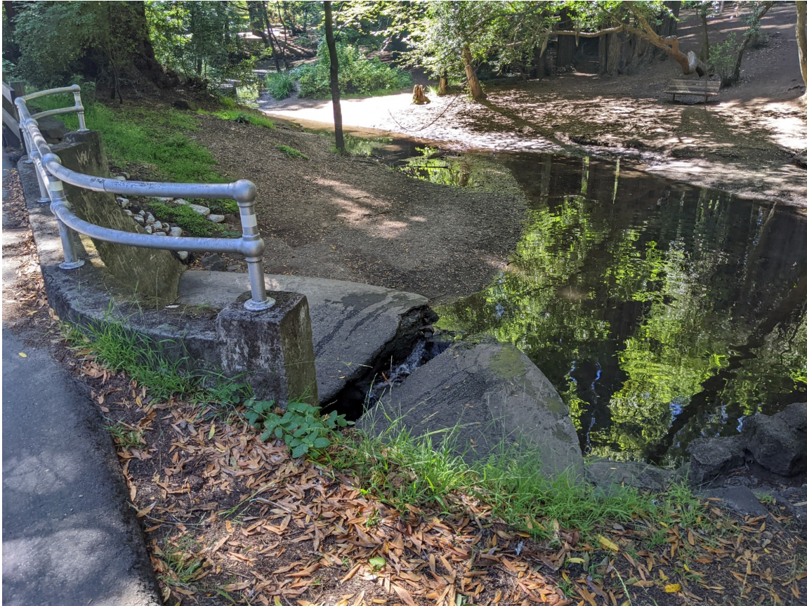
Looking upstream from Cascade Way roadway to creek and failing concrete-covered apron (June 15, 2022).
