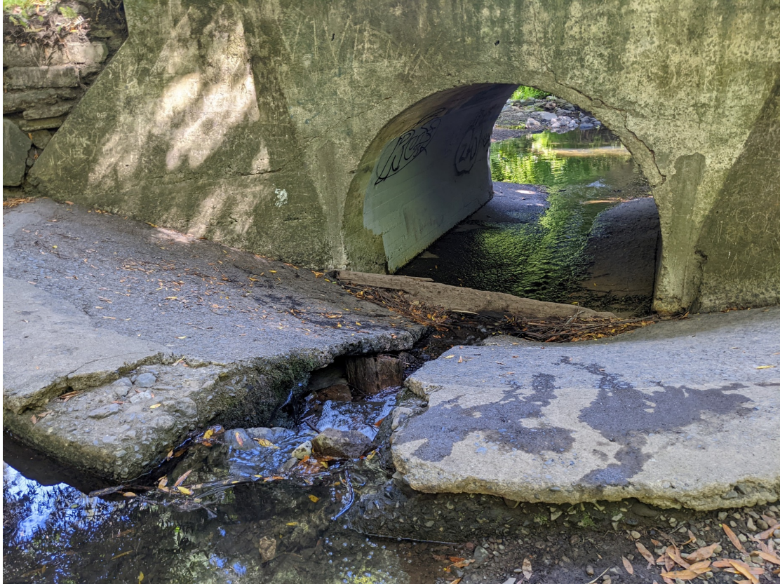
Looking downstream from top of concrete-covered fill apron through the culvert barrel (June 15, 2022).
